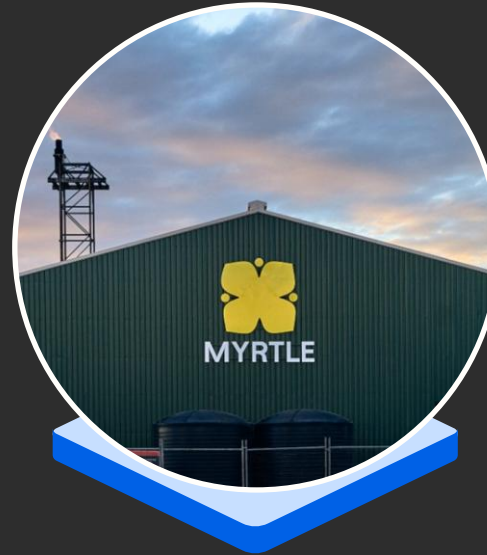
'Myrtle' Demonstration Plant
