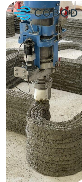
3D concrete printing
